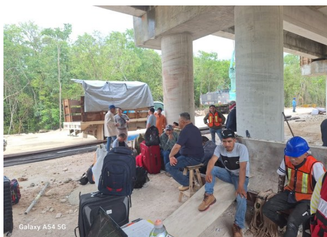
Construction personnel at the viaduct work front.
