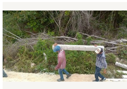
Transport to the work front.
