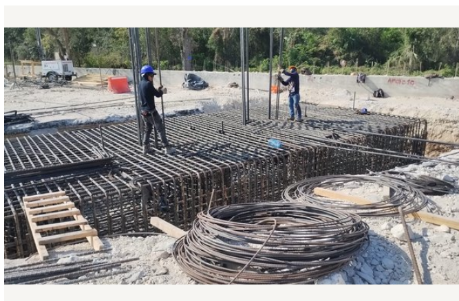
Reinforcing steel fabrication.
