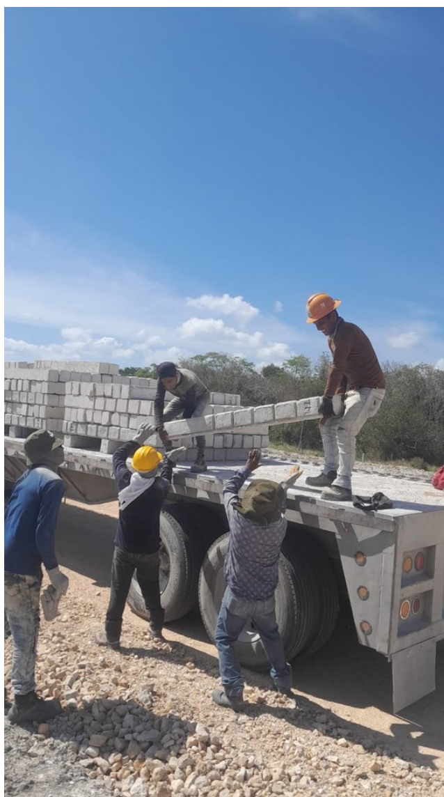
Unloading posts at the work front.
